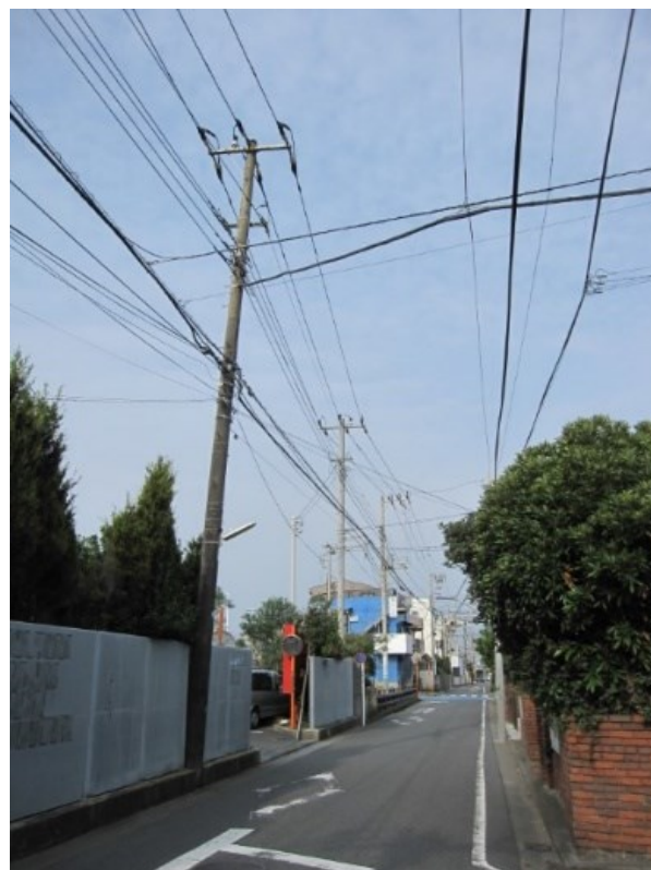
Photo 1.2 Overhead distribution line
