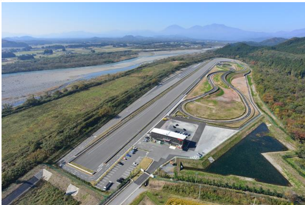
Fig. 6.32 Whole view of Showa Shioya proving ground
