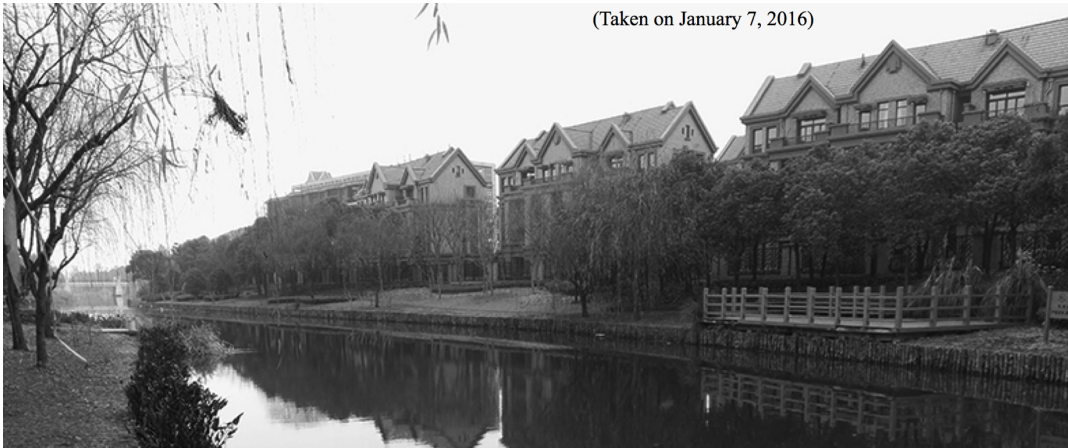
Figure 3-11 Revetment Constructed Along the Waterway
