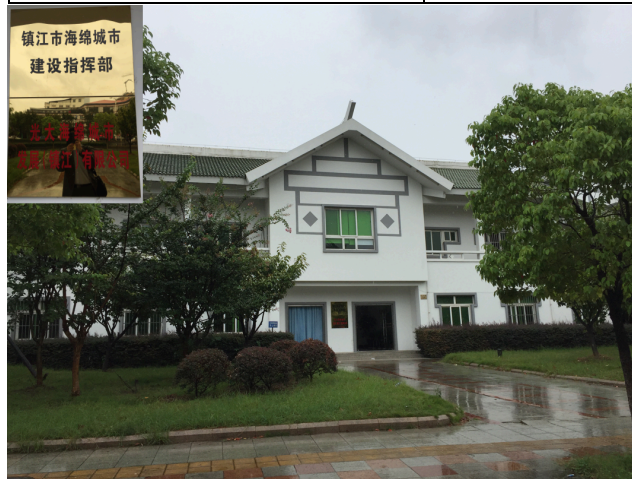
Figure 5-11 Zhenjiang Command Center for Sponge City Construction
