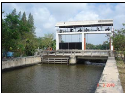
Figure 3.25 Sluice gates for regulating brine and fresh water flows
