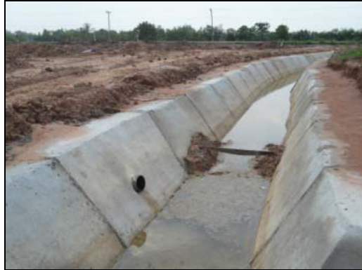
Figure 5.7 Drainage system for reclamation severely saline soil
