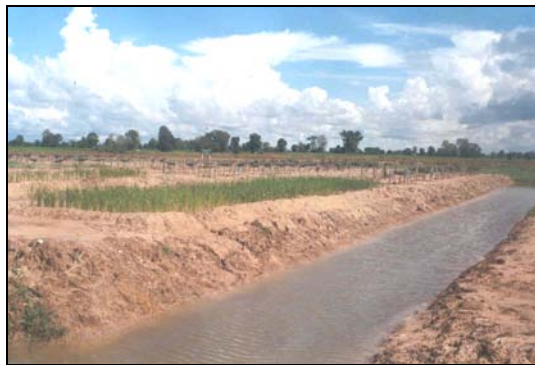
Figure 3.23 Open drainage system at Khon Kaen province, Thailand
