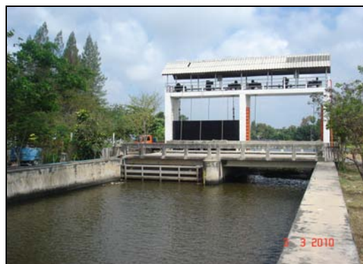
Figure 2.13 Dikes construction to prevent high tides
